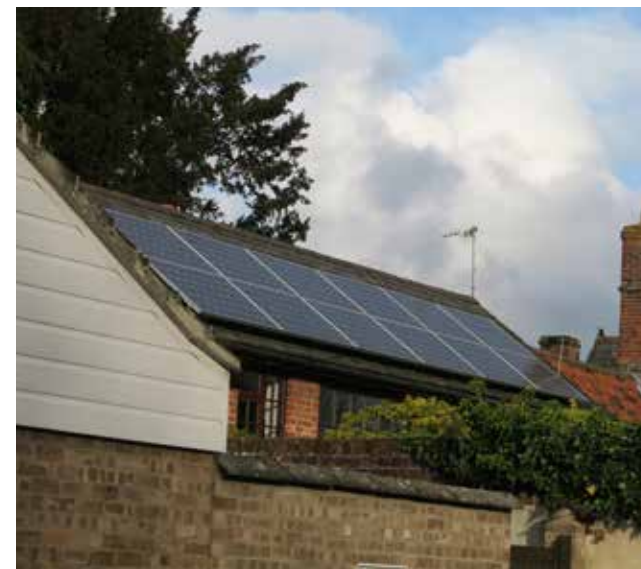
Figure 80: Existing building retrofitted with photovoltaic panels in Eye.
