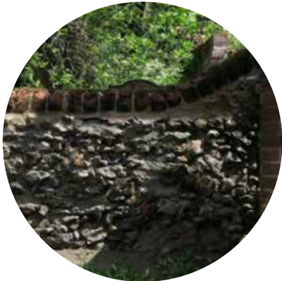
Pebble wall with red brick trim and cap
