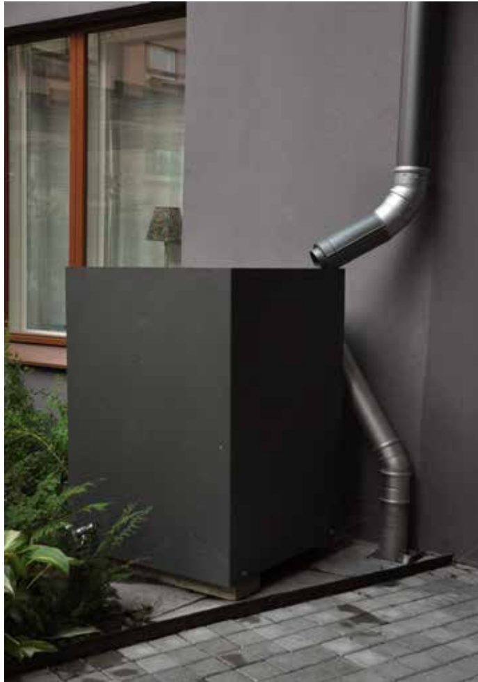
Figure 81: Examples of tanks used for rainwater harvesting © Wikimedia Commons (right).
